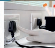
Electrical Switch Boards
